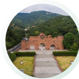
Everbright Bank supported the construction of the Huaguo Mountain Scenic Area in Lianyungang
