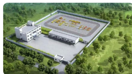
Distribution station of the natural gas pipeline project in Henan Province
